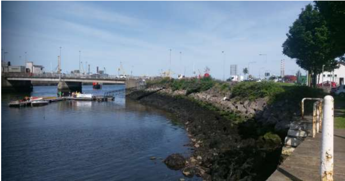
Photograph 1 Looking northwest towards Tom Clarke Bridge over the area which becomes reclaimed land.
