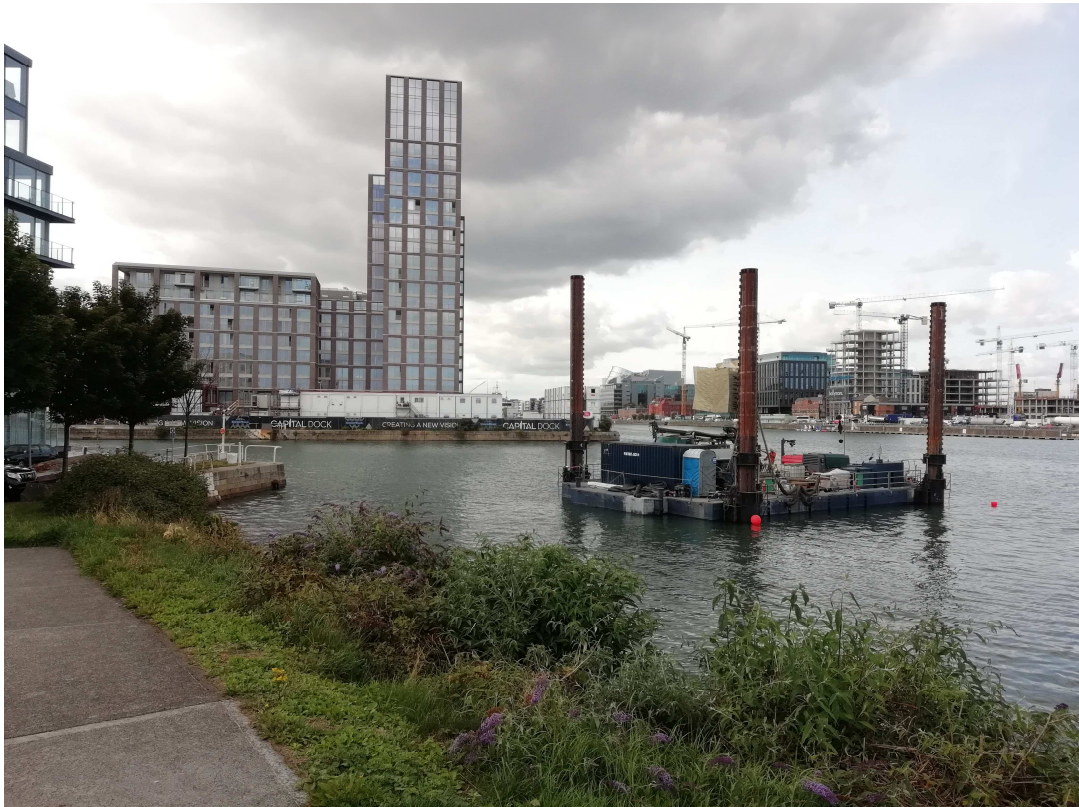
Figure 2 – Jack-up barge at Location 510
