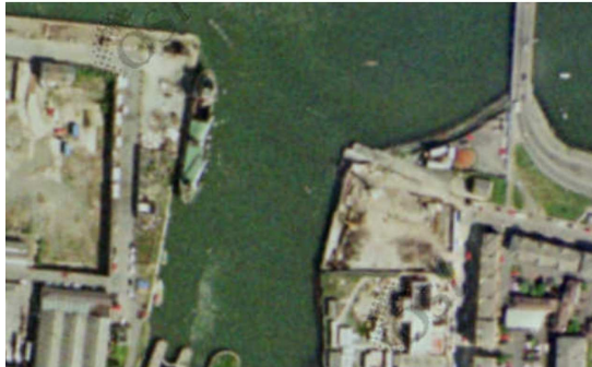
Figure 12D – Aerial Basemap 2000 orthophotography picturing the demolition of the existing warehousing at Thorncastle Street. A temporary site compound appears on the former green area at St Patrick’s Boat Club. Clearance work has removed all preexisting infrastructure at Britain Quay.
